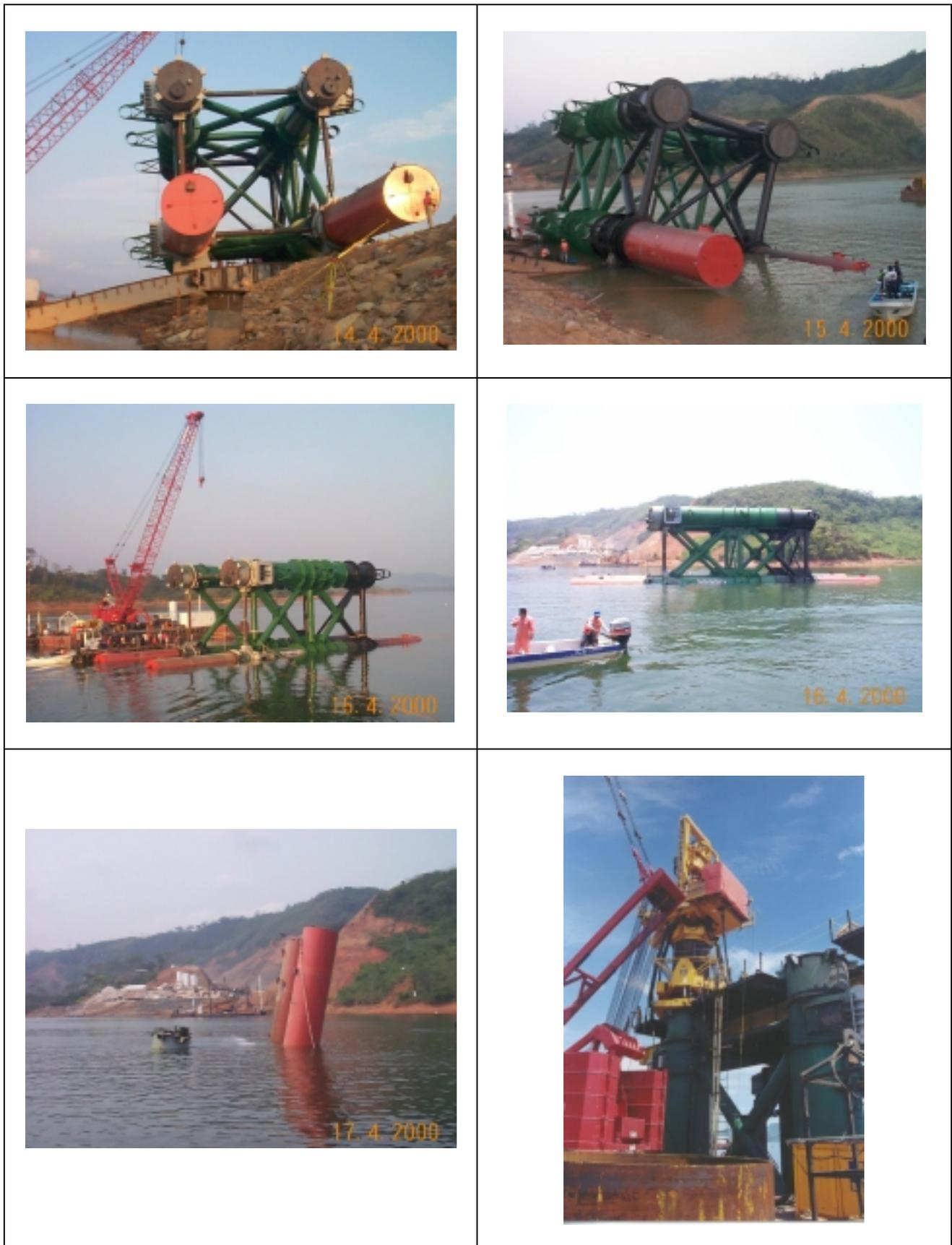
Fig. 7 Launching, transportation, positioning and drilling of pier (jacket) 8
