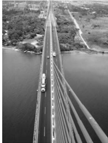
Figure 2. Example of traffic conditions on the A. Dovalí bridge used as ambient excitation.
