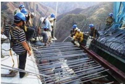
Fig. 18: Checking the target profile, before closing the main span
