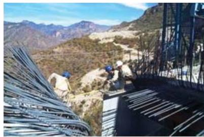
Fig. 19: Measuring of the last steel segment
