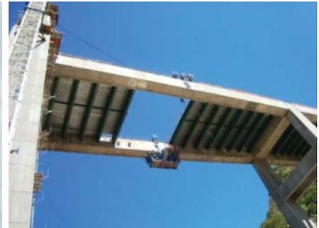
*Fig. 10: Closing of typical viaduct span*
