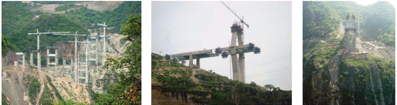
Fig. 5: Piers and Pylons during construction
