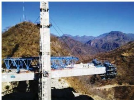
*Fig. 11: View of pylon 6. Ready for starting the construction of composite segments*
