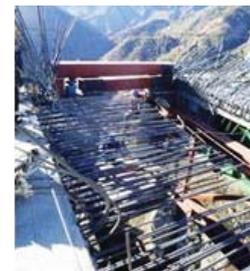
Fig. 20: Installation of a closing device to control thermal deformations
