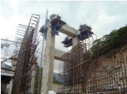
*Fig. 8: Steel reinforcement for concrete segments*
