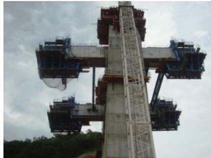
*Fig. 9: Construction of the double-cantilever*
