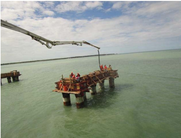
Figure 17. Cast of pile cap
