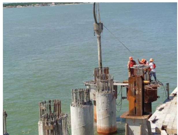
Figure 16. Cast of concrete in piles
