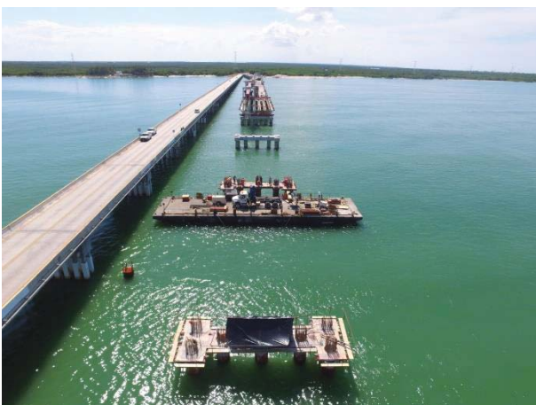
Figure 24. Aerial view of the construction works
