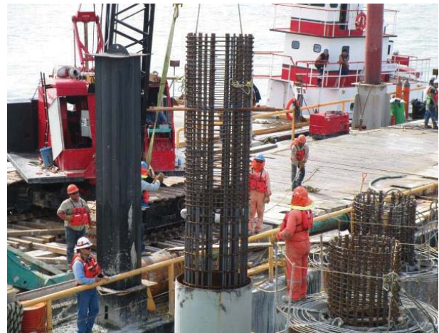
Figure 15. Installation of steel armature of piles
