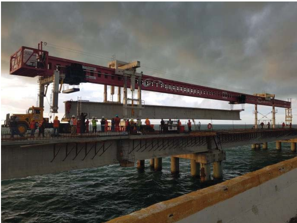
Figure 22. Installation of precast beam
