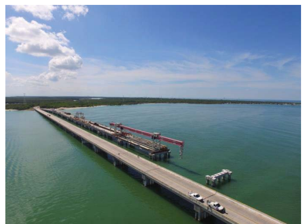
Figure 21. Aerial view of the launching gantry on the north side of the bridge
