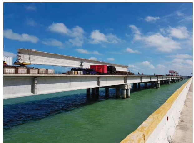
Figure 20. Circulation of a precast beam on the bridge
