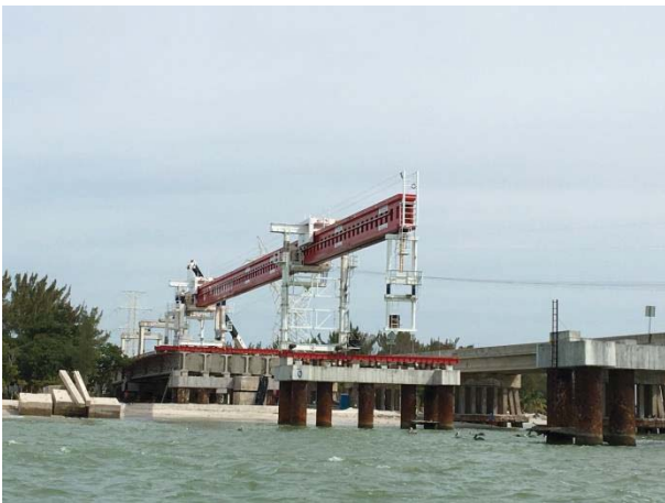
Figure 23. Launching gantry on the south side of the bridge
