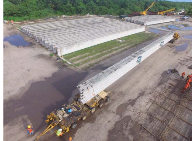
Figure 19. Precast beams manufacturing plant
