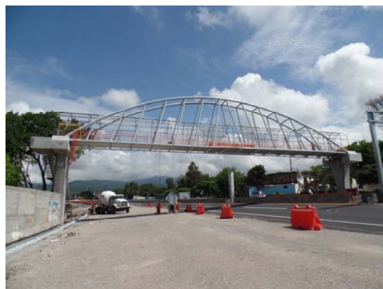
Fig.16. General view of one of the bridges during erection
