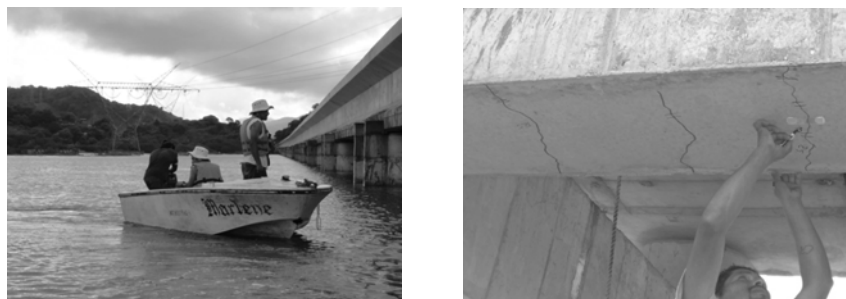
Figure 5 : Inspection work and detection of small cracks.
