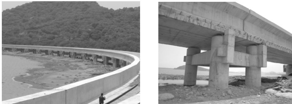
Figure 4 : General view of the deck and view of a typical pier
